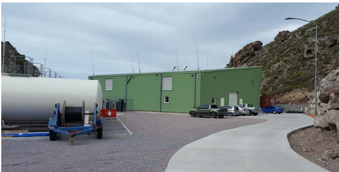
Figure 12: SEC new power plant
