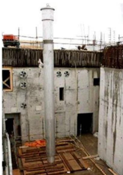
Figure A.4 Emplacement of wells during construction
