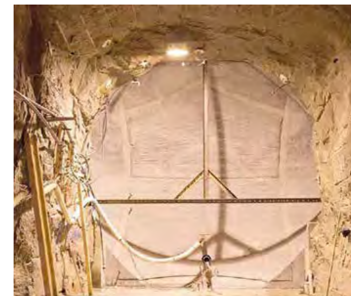
Figure 2-7: The cast concrete face of the composite DOMPLU test disposal tunnel plug at the Äspö URL in Sweden (image: SKB).
