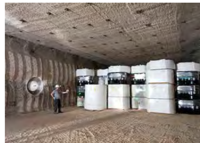
Figure 2-6: The WIPP facility in bedded salt formation in New Mexico, USA, for the disposal of defence transuranic and other wastes. This cavern has been excavated in the salt using conventional mining techniques.
