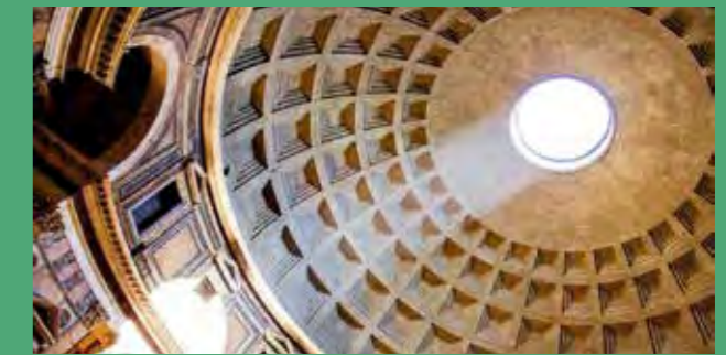
Above the unreinforced concrete dome of the Pantheon in Rome was built in about 120 AD and retains its structural, load-bearing integrity, 1900 years later.
