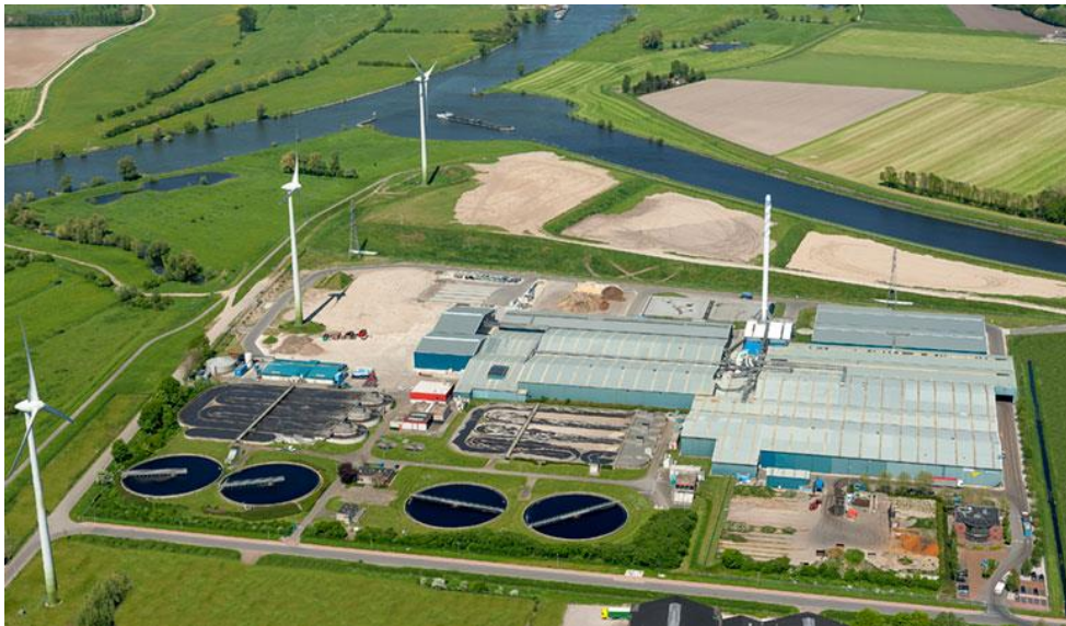
Figure 31: Wastewater and Sludge Processing Facilities in Zutphen
