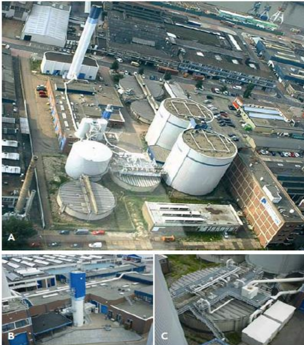
Figure 27: A) Sludge Treatment facilities in Dokhaven WWTP, B) View on Anammox, and C) SHARON Reactors
