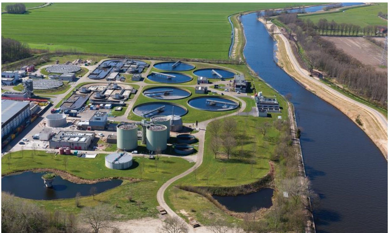
Figure 28: Energy and Nutrient factory at Amersfoort WWTP in The Netherlands
