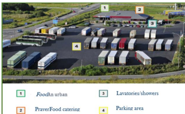
Truck Center (Source: AMDL)
