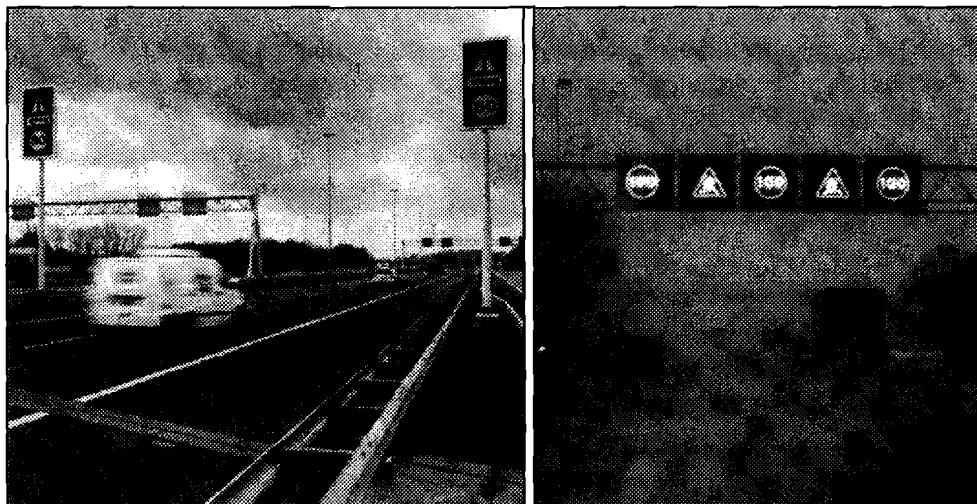
Figure 2 - Rotation signs indicate a lower speed limit due to poor air quality on the A58 (left); Overhead matrix signs on the A12 Bodegraven – Woerden show a speed limit of 100 km/h as imposed by the rain algorithm (right).
