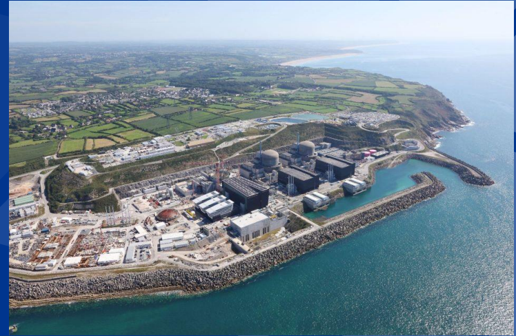
Fig 4: The Flamanville nuclear power plant in France( link )
