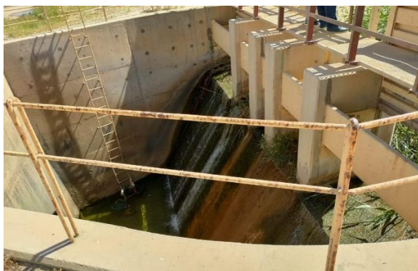
Picture 8. Picture of the sluice gate of the main irrigation canal of Hawija before IOM intervention. ©IOM, 2022
