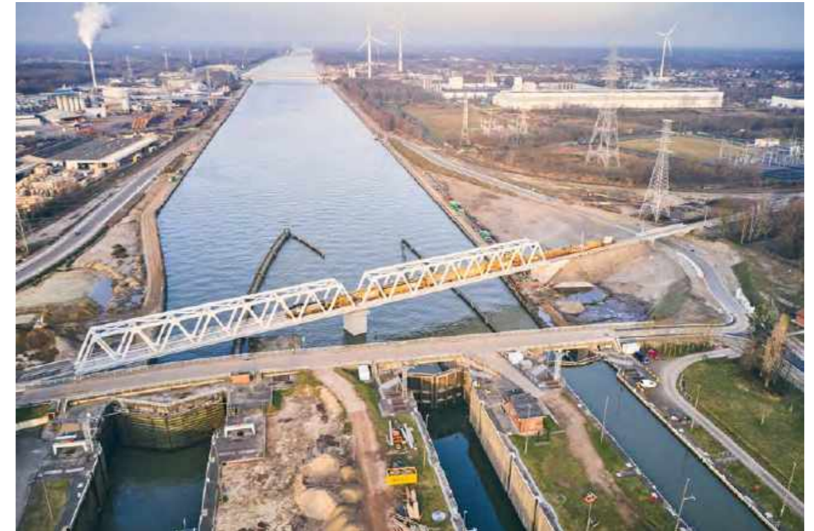
Construction works on the railway bridge crossing the Albert Canal near Genk.
