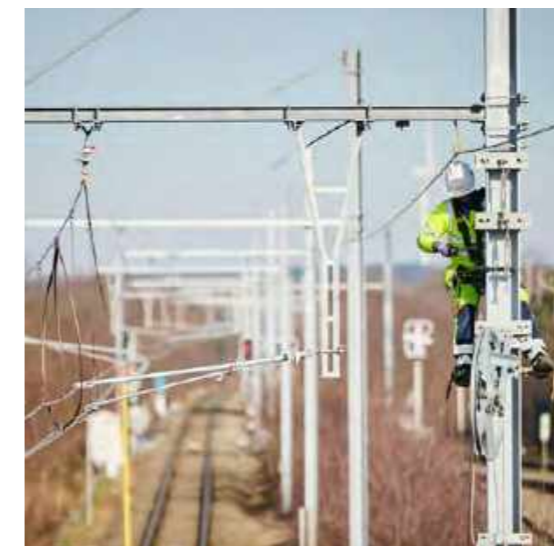
Electrification works between Genk-Goederen and Bilzen (L21C)
