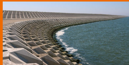
Financed as an eligible expenditure with the Dutch Green Bond, these Level-Blocs save up to 56% of CO 2 emissions in construction.
