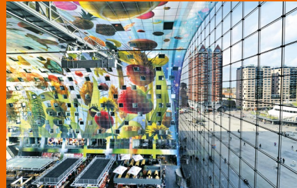
The Markthal in Rotterdam features the largest glass-window cable structure in Europe.
