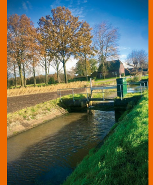
This classic sluice in the Brabant Delta near your my exemplifies the region's centuries-old water management practices, where early sluices and dikes were constructed to reclaim land from the sea and protect against flooding.
