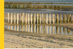
Breakwaters on the beach of Zoutelande (p. 9)
