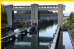
Lock in the Juliana Canal near Limmel (p. 26)
