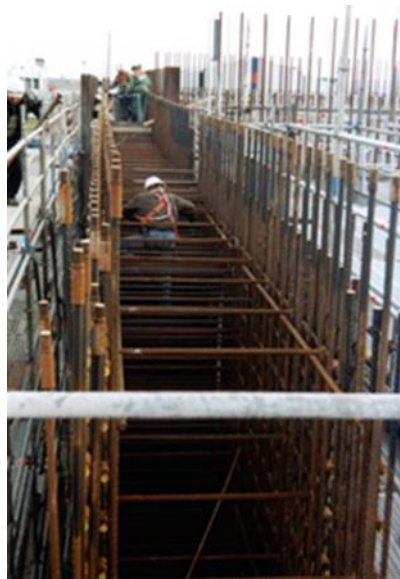
Figure A.5 Worker at work in a concrete 1.7 m thick outer wall
