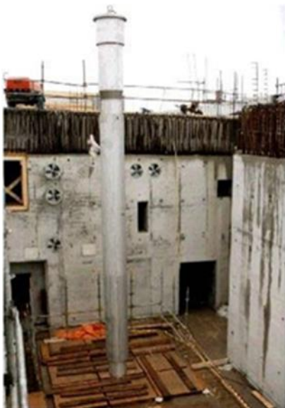
Figure A.4 Emplacement of wells during construction
