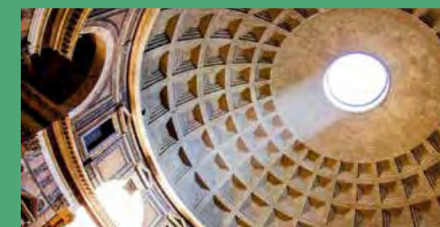
Above the unreinforced concrete dome of the Pantheon in Rome was built in about 120 AD and retains its structural, load-bearing integrity, 1900 years later.
