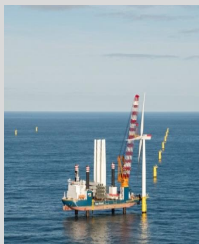
Van Oord at work at Gemini Wind Park
