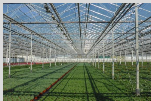
Geothermal energy in the Netherlands is mainly used for greenhouses
