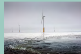
Princess Amalia windturbine park on the North Sea, twelve nautical miles from IJmuiden (p 30)
