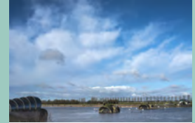
The 'balgstuw' (inflatable dam) near Ramspol protects against high tides from the Ketelmeer (p 38)
