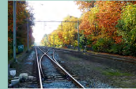
Dutch rail infrastructure in the fall (p 25)
