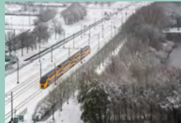
Aerial footage of Dutch rail infrastructure in winter (p 22)
