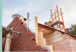
The construction of new housing with an emphasis on insulation (p 15)
