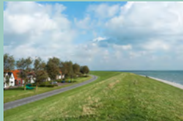
Reinforcing the dikes on the island of Texel to protect the village of Oudeschild (p 12)
