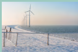
The IJsselmeer dike with wind turbines in a snow landscape (p 1)
