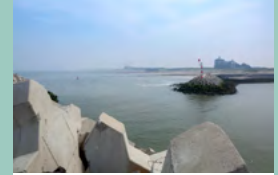
Innovative ways to reinforce dikes and sea barriers near Cadzand (p 33)
