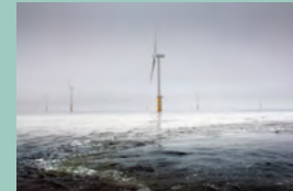
Princess Amalia windturbine park on the North Sea, twelve nautical miles from IJmuiden (p 30)
