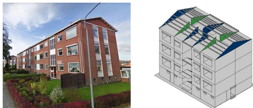
Figure A.16 Rijksweg 119-129, Delfzijl: side view (left, taken from Google Street View) and corresponding FEM model (right) adopted in [VIIA 2019b].
