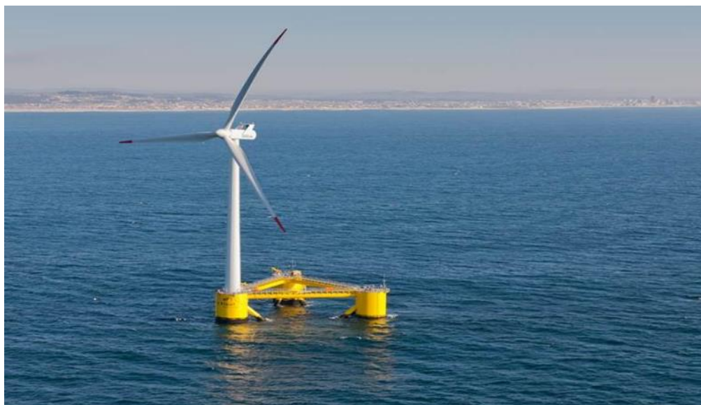
The Windfloat project, Portugal
