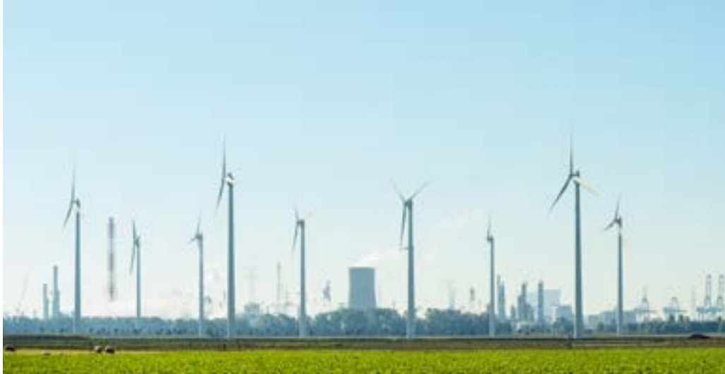
Windpark Rilland in Zeeland.
