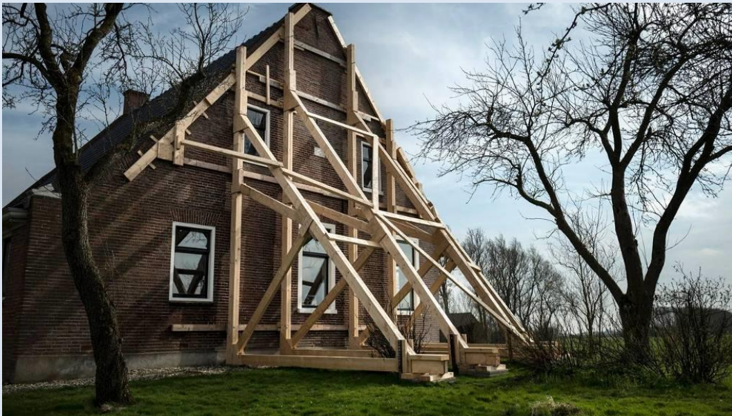
Schade door aardgaswinning [57]
