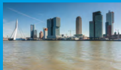
The tallest buildings in the country in Rotterdam (p. 11)
