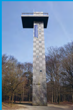
Watch-tower De Kaap near Doorn (p. 10)
