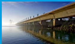
Eastern Scheldt storm surge barrier (p. 5)
