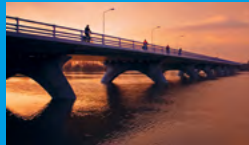
Bridge over the river forelands of the Rhine (p. 8)
