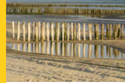
Breakwaters on the beach of Zoutelande (p. 9)
