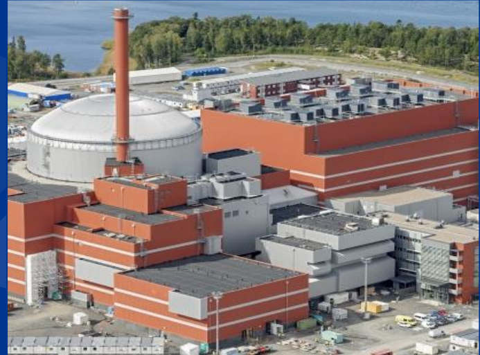
Fig 2: Olkiluoto Nuclear Power Plant Unit 3 Project ( link )
