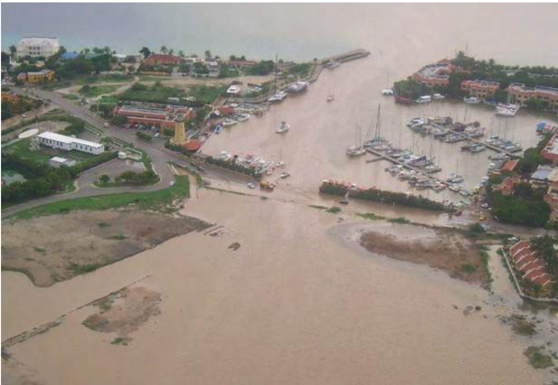
Figure 3.2 Overflow of the saliñas following intense rainfall. Flooding causes sedimentation in the built environment
