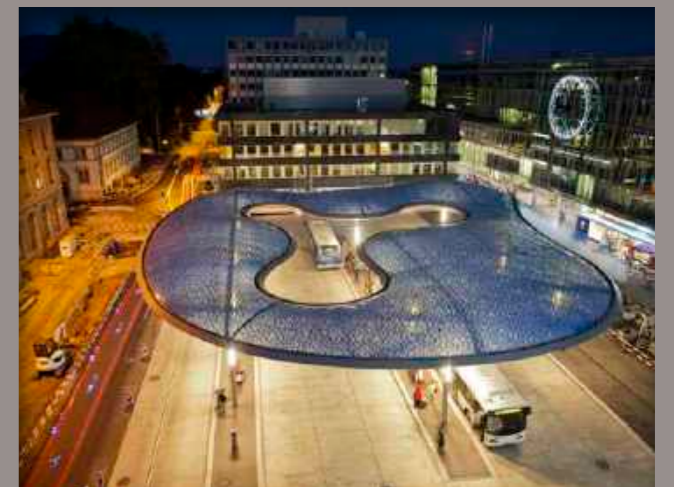
4. Aarau Bus Station canopy
