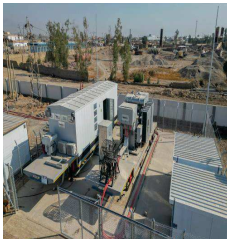
View showing the mobile substation in Hawija, installed.
